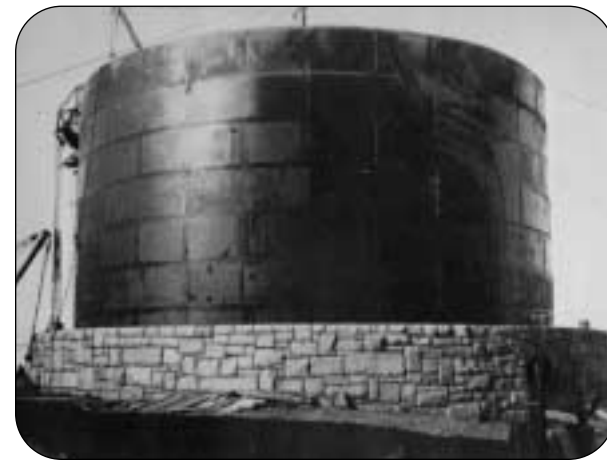
Top: The Thomas Hill Standpipe today. (NEWS Photo by David M. Fitzpatrick.) Right: The 1.75-million-gallon Standpipe under construction in 1897. The inner steel structure is visible here. The project, employing 22 men, took six months to complete.
