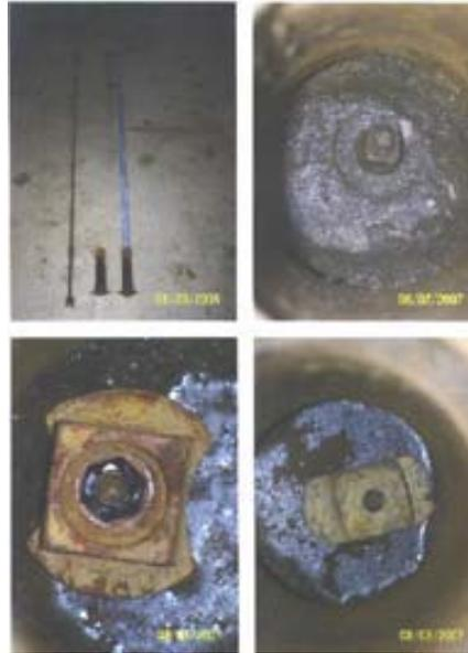
**1<sup>st</sup> Place** winner was Cam Torrey of Hampden Water District for his Valve Stem Rethread (New Operating Nut) Tool. Total cost to build estimated at \$48.00. HWD figures they saved \$1,000-2,000 last year alone by not having to excavate valves when replacing rounded or worn gate valve operating nuts.
