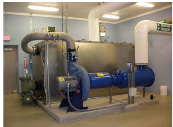
Madawaska Water District New Pump Station and Aeration Facility
