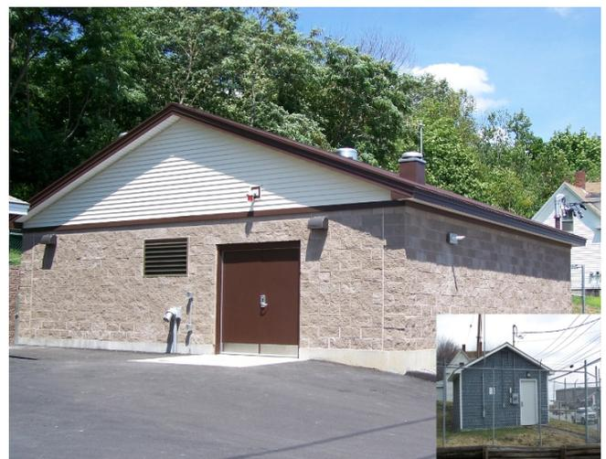
*"The Hampden Water District has rebuilt the antiquated 1960's Pump Station into a state of the art pump station and treatment facility. Some changes in our system, since being put into operation in May 2010, are the addition of soda ash to combat our lead leaching issue in older homes along with the addition of carbon dioxide to reduce our pH levels.*
